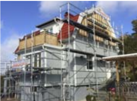
Kaycan PVC fasad under montering.
